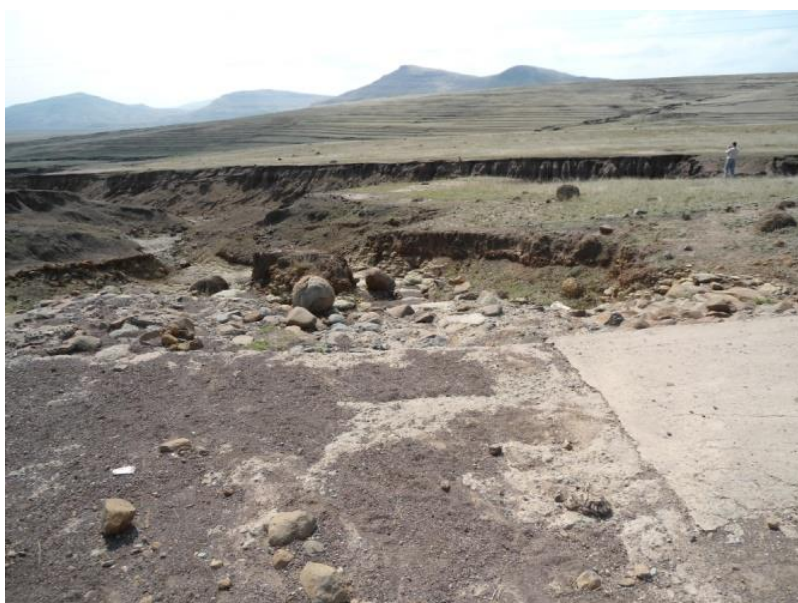
Figure A-5: Donga Erosion Occurs in Many Stream Channel Sections
